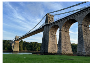
Famous Bridge in Bangor Called "Menai Bridge"
